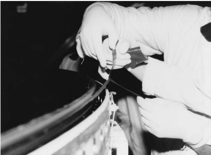
Figure 2 A risk-taking culture? This 1985 photo, which I found at the NASA Photo Archives, Washington DC, shows two NASA technicians dressed in surgical scrubs using antiseptic tape to inspect and place an O-ring in its groove in a Solid Rocket Booster joint.
